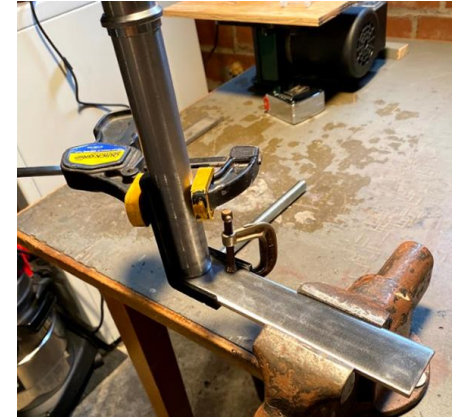
Welding the Kingpins
