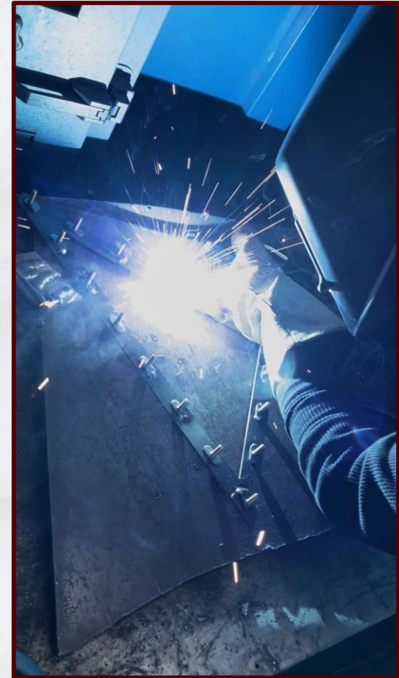
Figure 36. David welding plate nuts to inside of reservoir port
