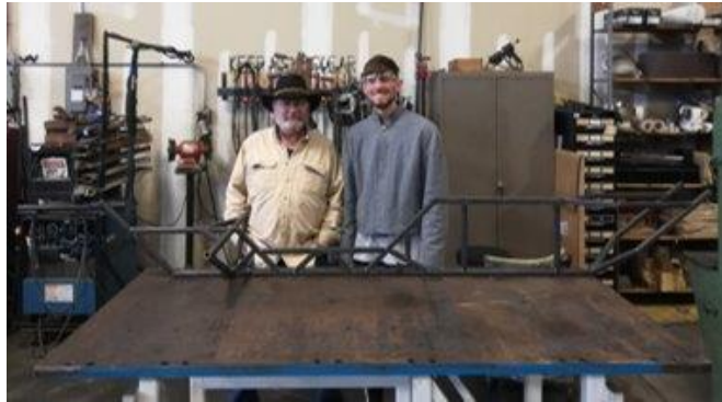
Tack welded the main frame
