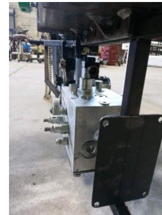
Mounting Manifold and controller to the frame
